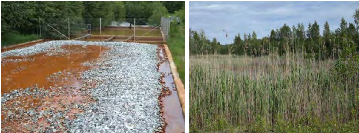
Figure 26. Water treatment plant based on limestone buffering in the closed Kotalahti mine area (left). Vegetation is well distributed in the tailings waste area, forming wetlands suitable for metal binding (right), Leppävirta, North Savo. (© A. Tornivaara, GTK)
